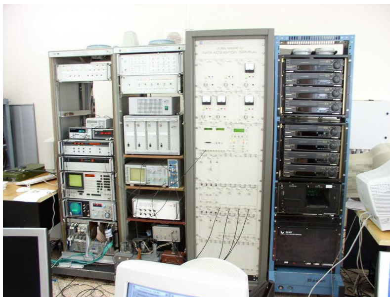
Figure 1. VLBI Data Acquisition and Recorder Equipment at Zelenchukskaya observatory
