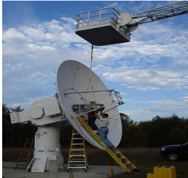
Figure 1. Installation of new wide band dewar on MV3 antenna.
