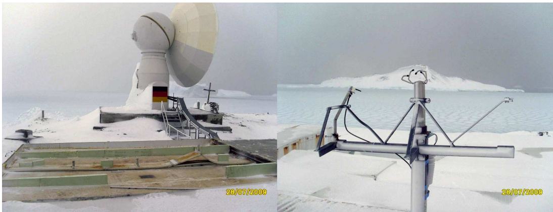
Figure 3. The destructions caused by a strong storm: unroofed containers and a totally damaged meteorological site
