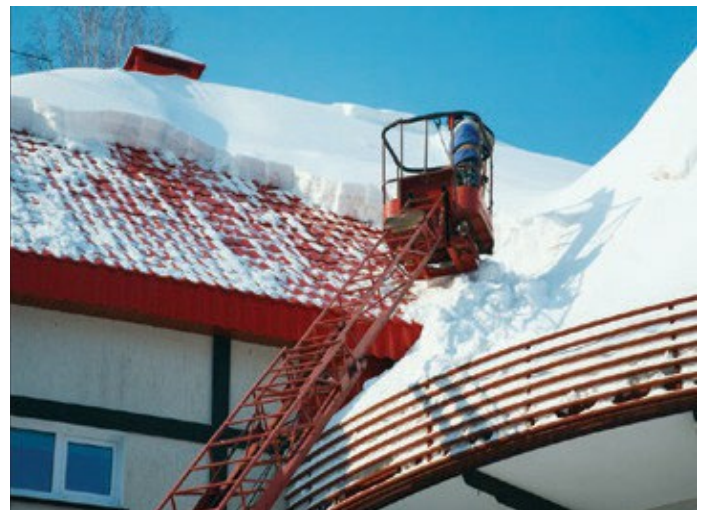
An aerial lift is being used in a snow removal operation. The worker is using a restraining belt and lanyard for protection.
