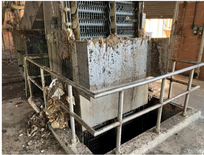
Image 1: IPI Building, Screen 2.
