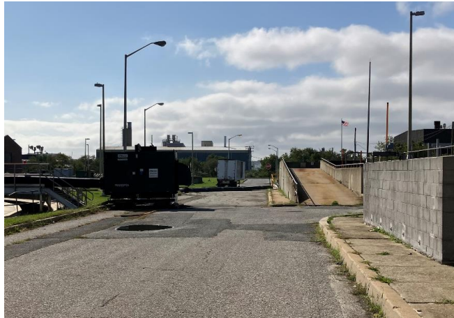
Image 4: United Rental Pump area.
