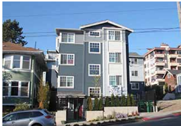
This micro-housing complex at 1304 E John St has 56 studios.
