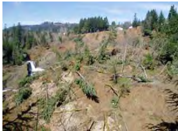
Piper Road Landslide, 2007, Photograph by Larry Douglass
