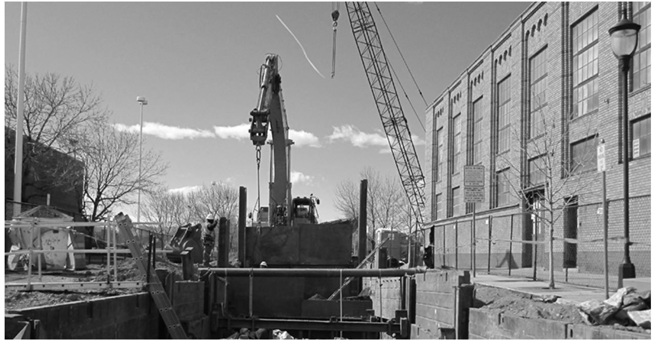
Dakota Outfall under construction from D4
