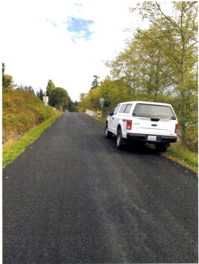
Concrete barriers MP 0.82
