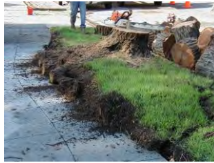
Tree failed in storm; was root Pruned
