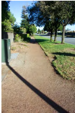
Decomposed Granite walkway
