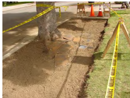
Sunnyvale, CA steel plates over roots
