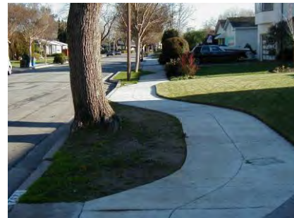
3 different sidewalk treatments; move away from tree, move sidewalk next to curb, move both sidewalk and curb away
