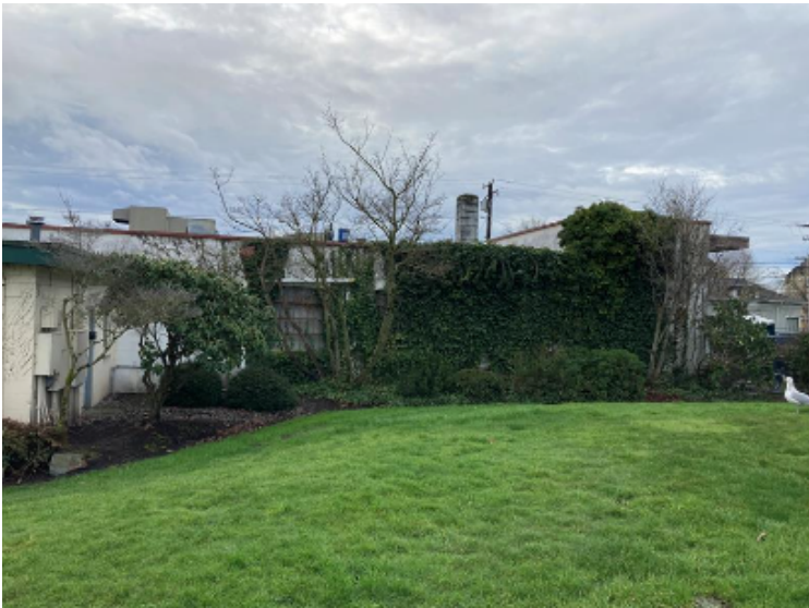
Vegetation to be removed
