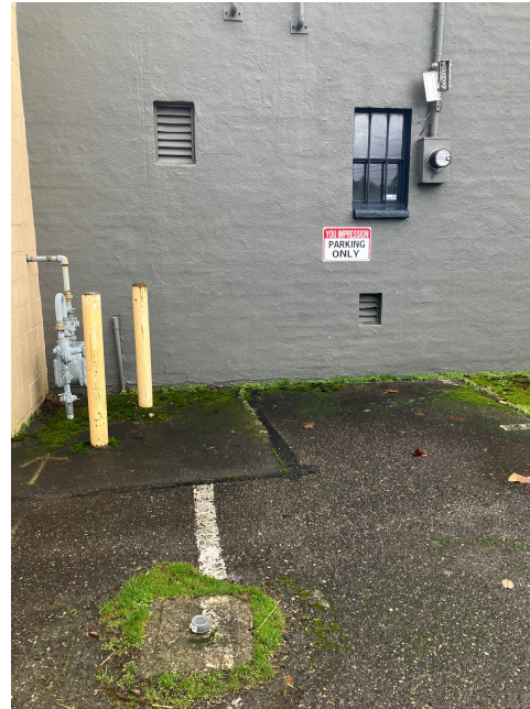
Underground tank to be decommissioned and removed
