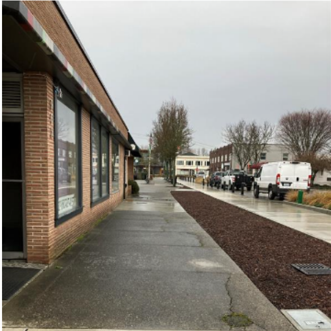
Sidewalk to be demolished
