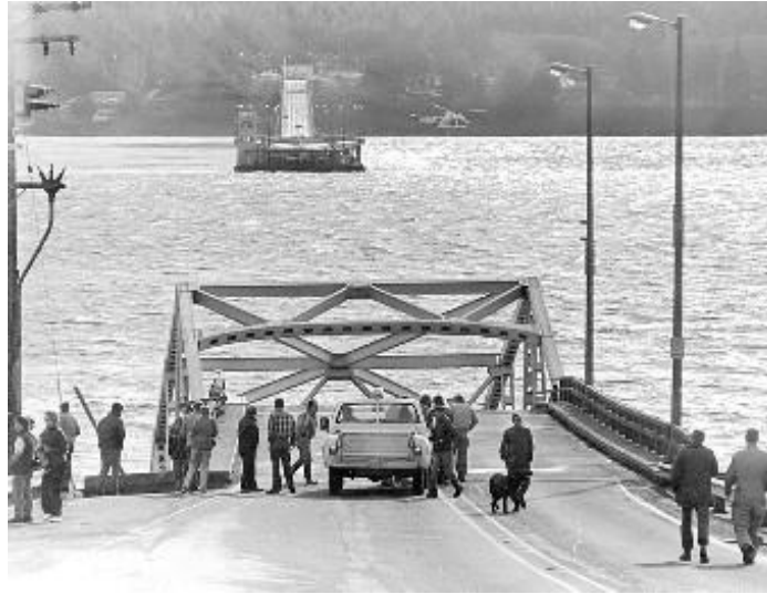
Hood Canal Bridge shortly after collapse 1979
