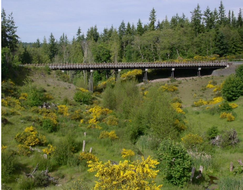
Bridge on Old Gardiner Road – rebuilt under the FEMA disaster assistance program after old bridge was destroyed by flooding.
