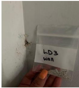
Laundry room wall
