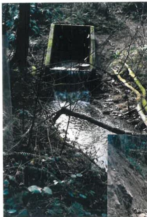
Figure 12. Adjustable channel of First Creek (Cosmopolitan Engineers, 1997).
