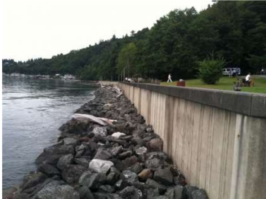
Figure 35. Seahurst Park Seawall in Burien. Photo credit: John Ryan / KUOW [267]
