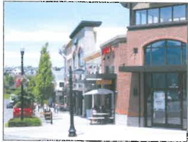
Part of the recent mixed-use development in the City of Snoqualmie, at the corner of Center Blvd SE and Mayrand Lane SE
