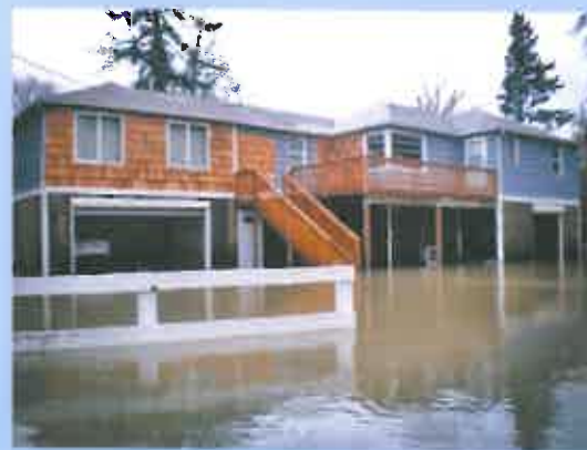
Elevated Snoqualmie Home - Living areas now protected from floodwater.
