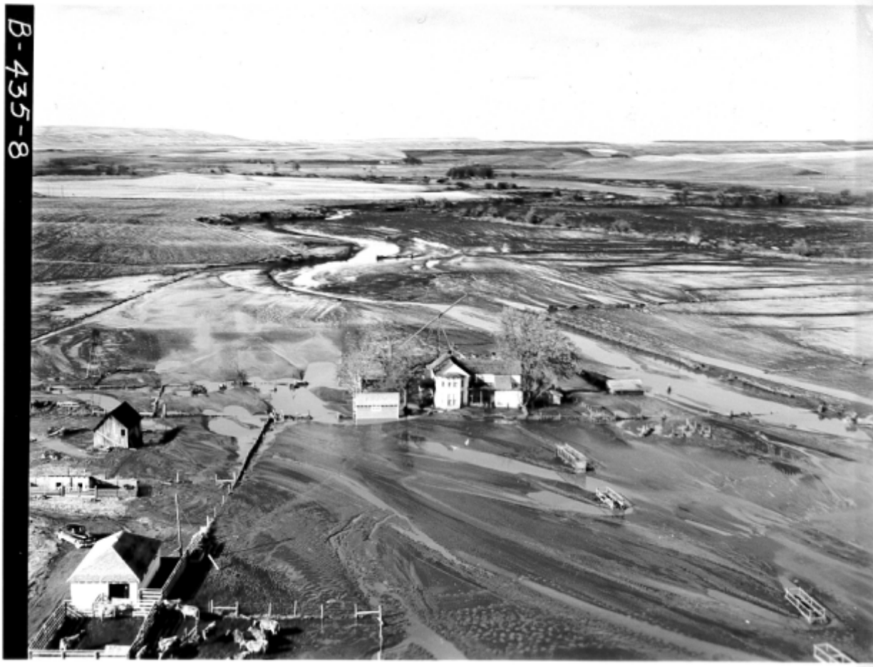
This is a USDA SCS flooding picture.
