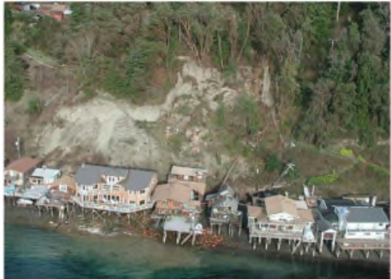
Figure 12. Salmon Beach, Tacoma, WA following Feb. 2001 Earthquake
