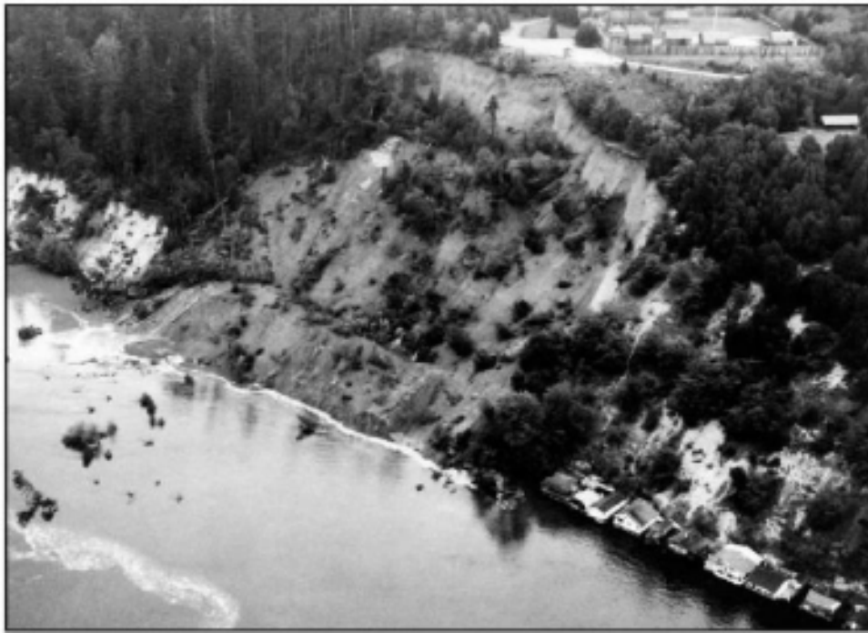
Figure 6. Salmon Beach, Pierce County, 1949--Tsunami Causing Landslide 10
