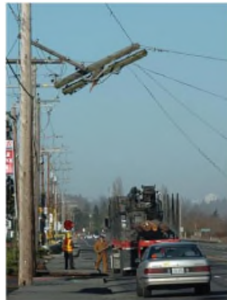
Figure 11. Impacts to Property and Infrastructure
