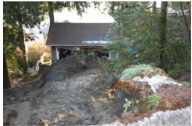
Figure 2. Home Damaged by Landslide during January 2012
