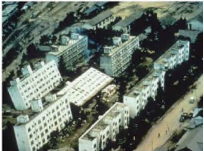
Figure 13. Liquefaction, Niigata Japan, 1964.
