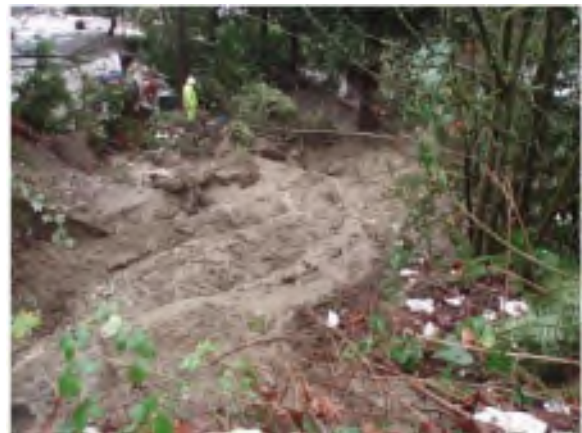
Figure 4. Hillside and Vegetation Damaged after Landslide in January 2012
