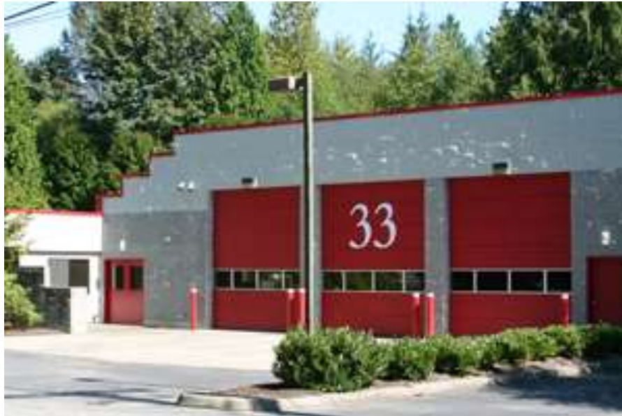
Survey Table 10: Woodinville Station 33 - 19401 NE 133rd St.
