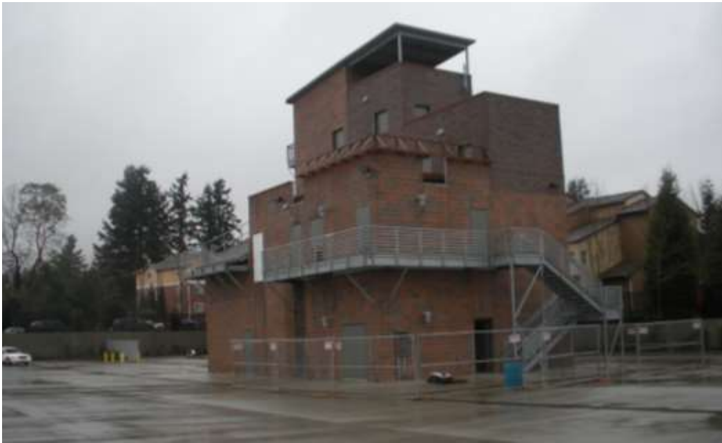
Survey Table 7: Training Tower Located at Station 51, Northshore
