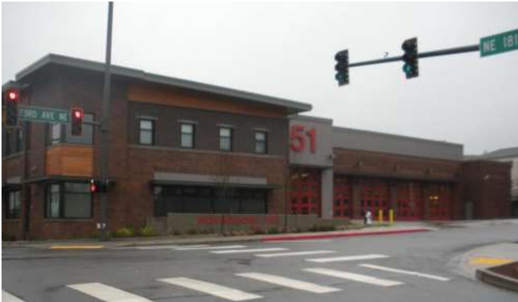
Survey Table 5: Northshore Station #51 - 7220 NE 181st Street, Kenmore
