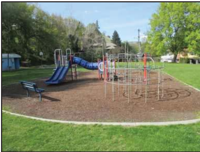
Figure 28. Newly installed playground equipment.
