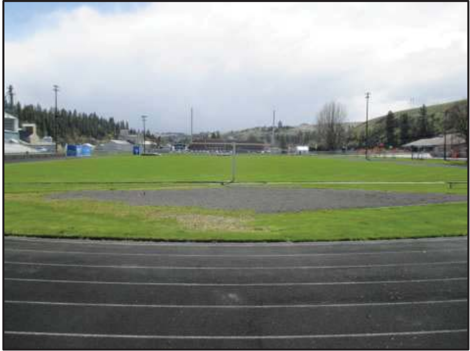
Figure 52. High school track in need of replacement.
