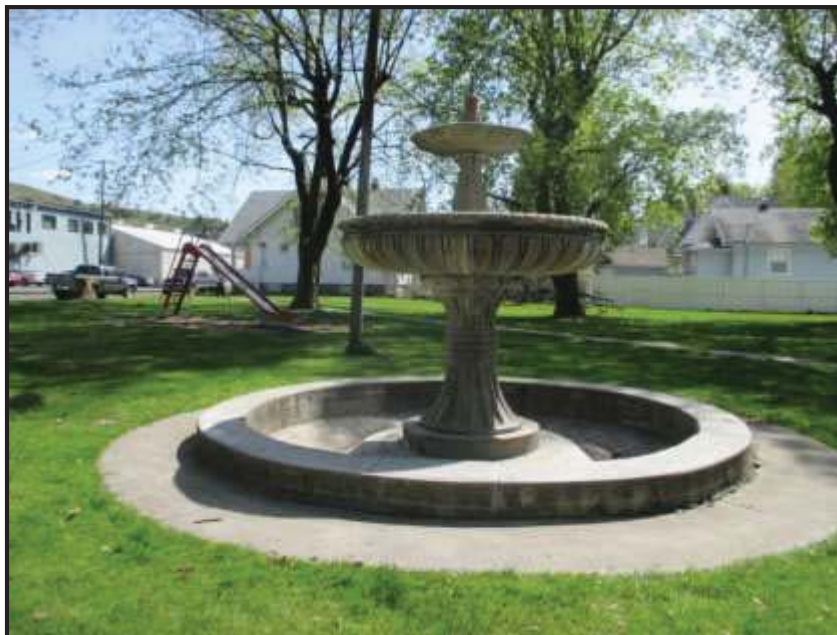
Figure 37. Water fountain monument (currently needing repair).
