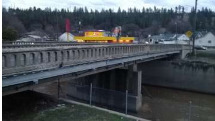
Image 18: State Route 26 Spur Bridge
