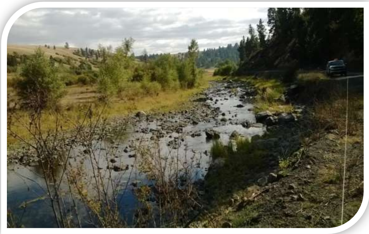
Image 1: Glenwood Water Line & North Palouse River Rd Area
