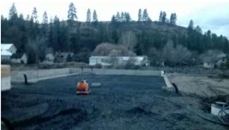
Image 63: Construction Work at Riverside Terrace Subdivision
