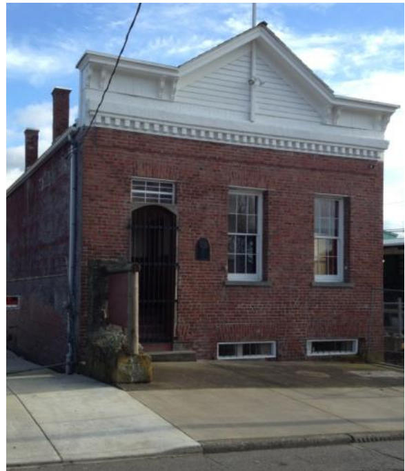
The Territorial Courthouse in Bellingham's Old Town is the oldest brick building in Washington State. (Photo courtesy Whatcom County Historical Society website.)
