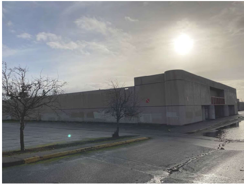
NORTHWEST BUILDING CORNER
