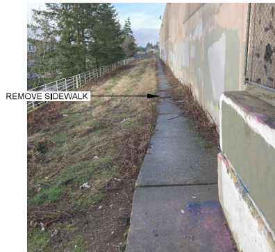
SOUTH SIDE WALKWAY REMOVAL
