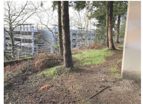
SOUTHEAST CORNER, WALL & RAILING
