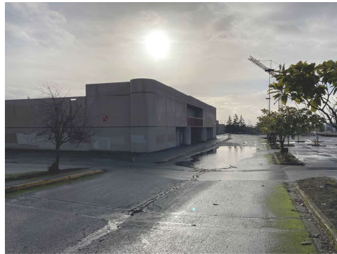
MAIN DRIVE AISLE
