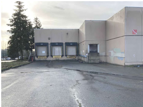
NORTHEAST LOADING DOCK
