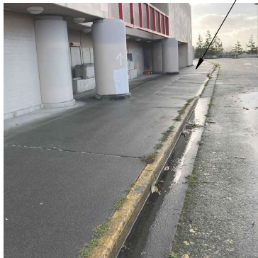
WEST SIDE WALKWAY REMOVAL
