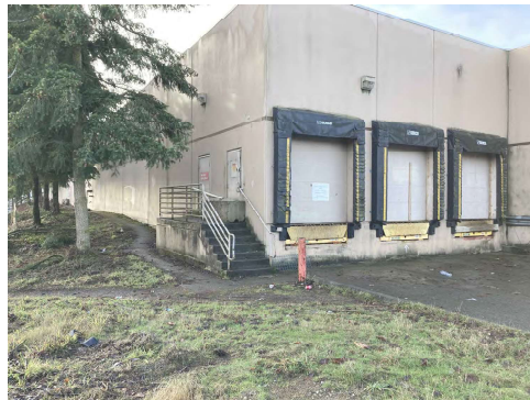
NORTHEAST BUILDING CORNER
