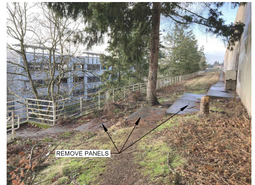
SOUTHEAST WALKWAY REMOVAL
