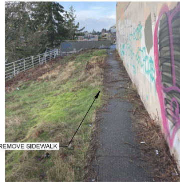
SOUTH SIDE BUILDING (FACING WEST)
