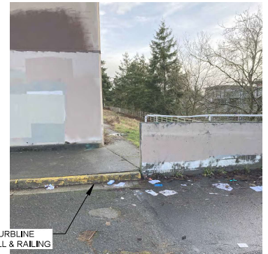
SOUTHWEST CORNER, WALL & RAILING
