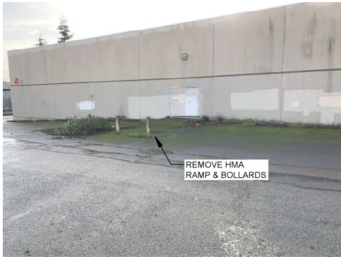
NORTH HMA RAMP REMOVAL
