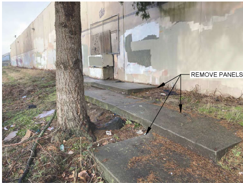
SOUTHEAST WALKWAY REMOVAL
