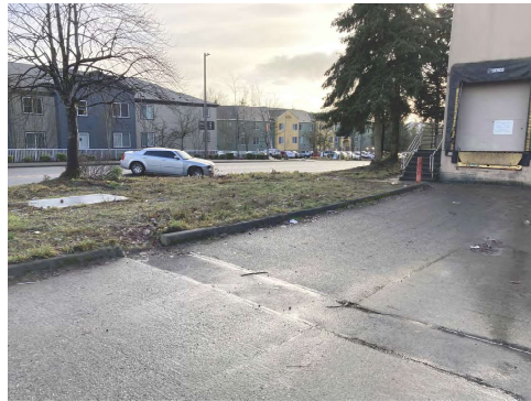
NORTHEAST POWER VAULT
