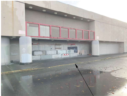
WEST SIDE BUILDING
