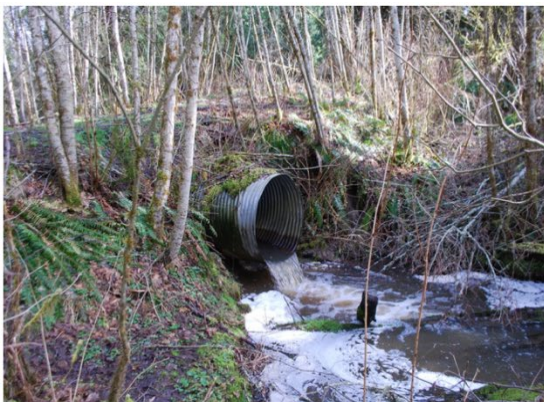
No migration – fish stuck below the culvert restored!
