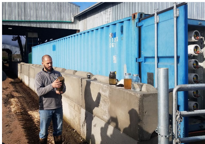
Figure 3.14: Coldstream Dairy Farm has installed a three-stage processing system to manage dairy manure and produce water clean enough to be returned to nearby streams.
