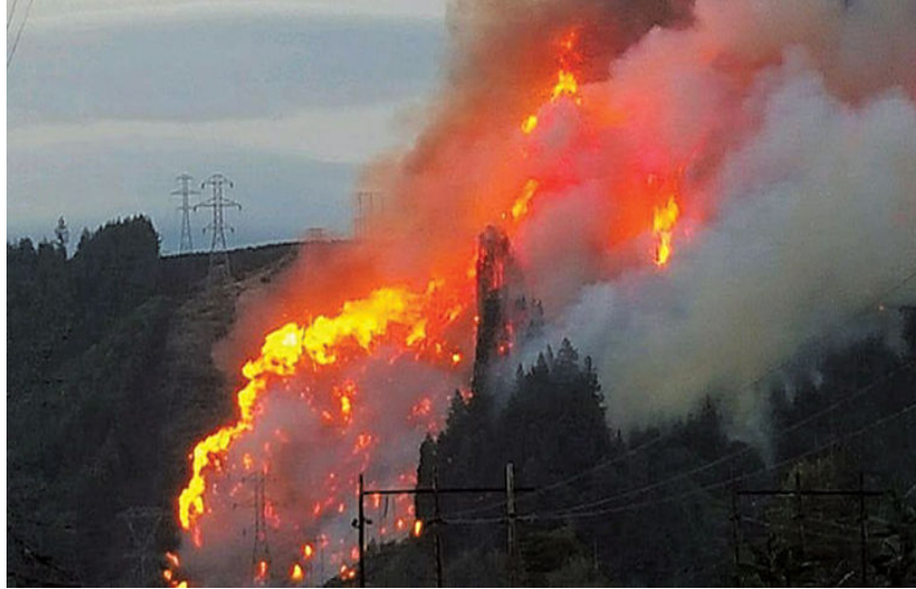
09/02/2015 Fire in Mason County Cuts Electric Service to Over 2000 Jefferson County Customers.
