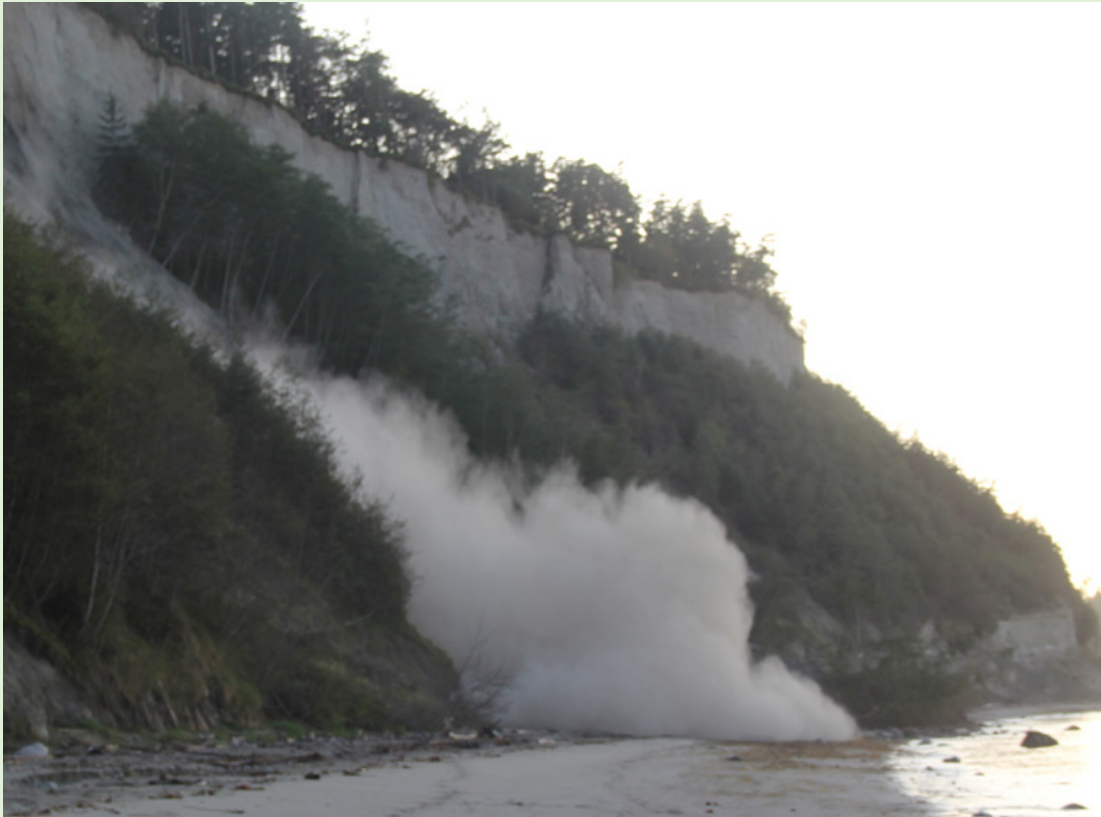
On Sunday, Oct. 13, 2013 another large chunk of sand and debris tumbled to the beach below “End of the World,” a bluff overlooking the Strait of Juan de Fuca on the edge of Port Townsend. Photo by Scott Wilson 17
