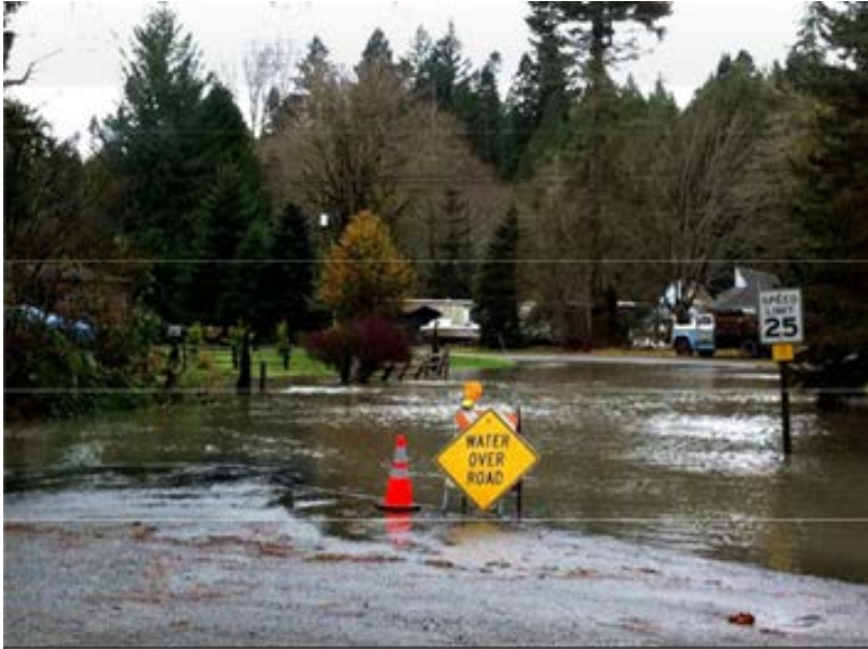
Kelly Road, Brinnon. 2010 Flooding. Photo by Julian Ray
