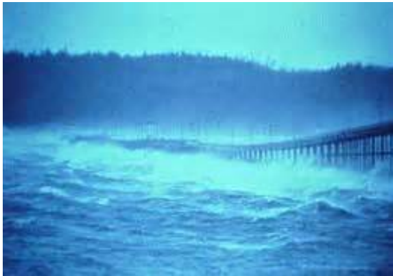
Hood Canal Bridge in a Windstorm. Unknown Date
