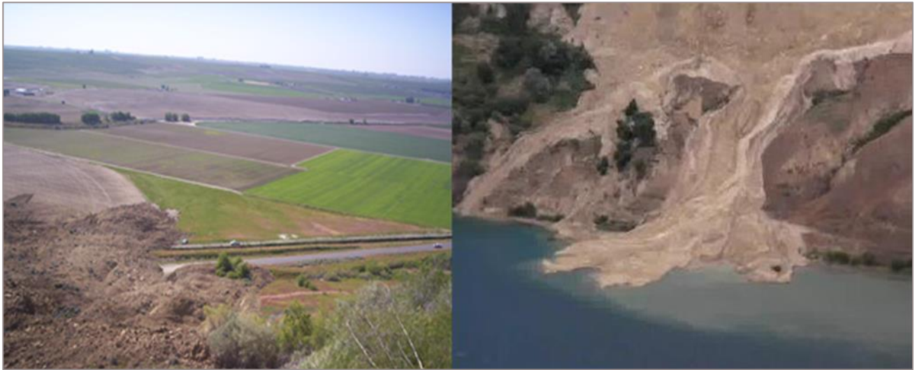
Figure 6: 2006 Road 170 Landslide (left); and August 2008 Columbia River Landslide (right).
