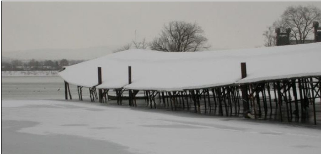
Figure 26: Pasco Marina damage from 2017 winter storm.
