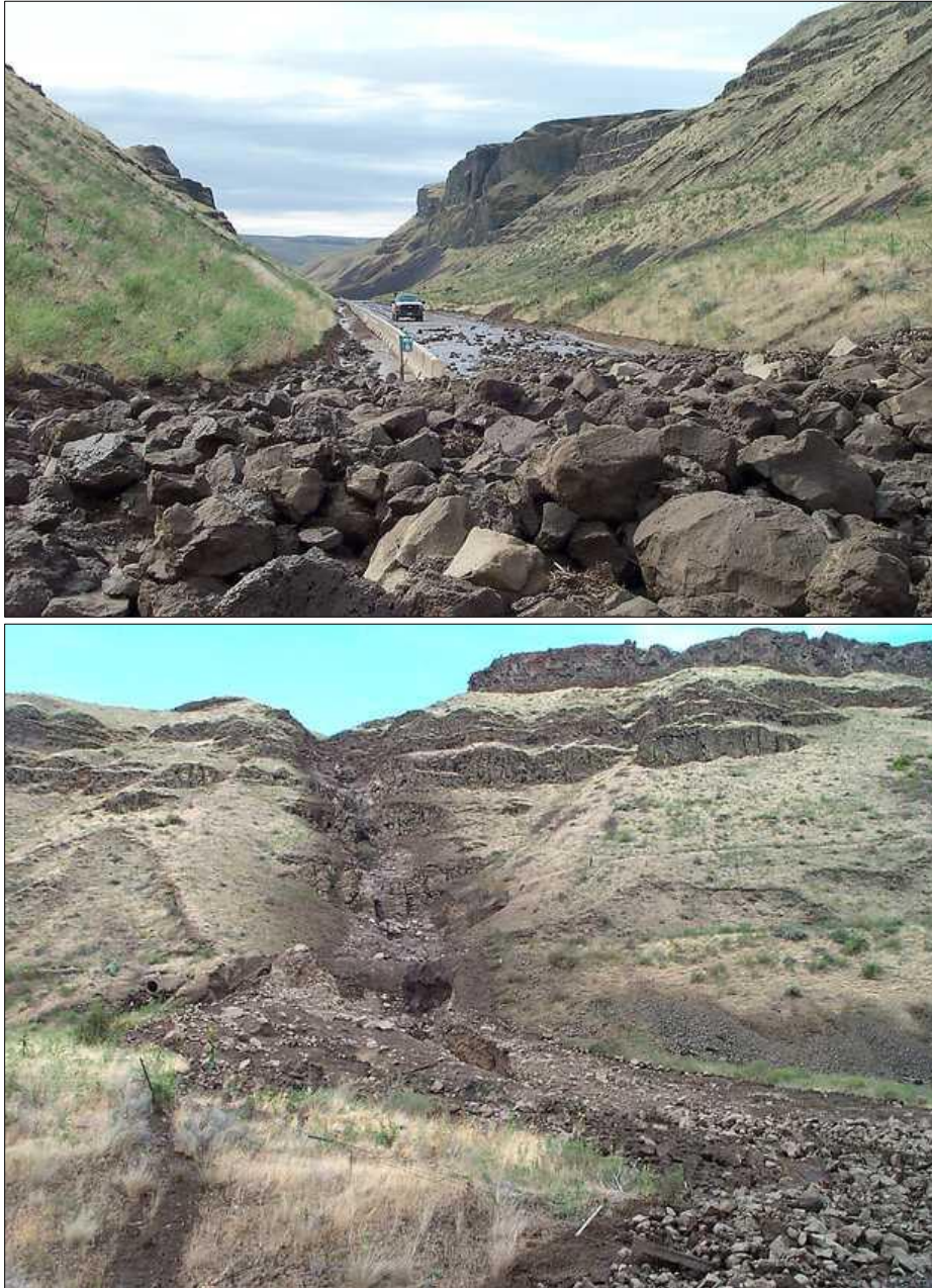
Figure 24: Rock slide on Pasco-Kahlotus Highway 07/16/12
