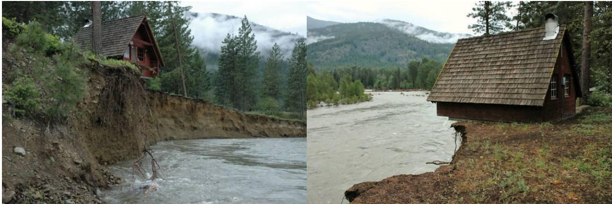
Figure 5.4. 2006 Landslide due to Flash Flooding in Methow River Valley.
