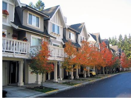
Townhouses along a private internal drive in Redmond. Source: MAKERS
