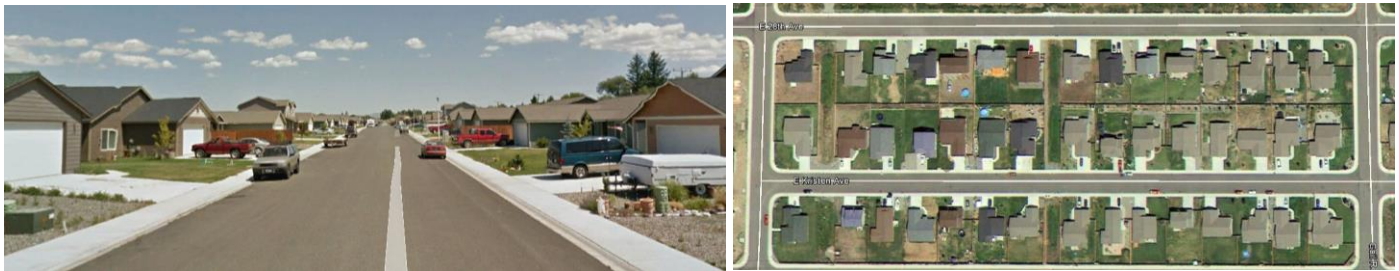
9.3 dwelling units per acre (gross) - Mixed-housing-type subdivision within the master-planned Issaquah Highlands development in Issaquah
