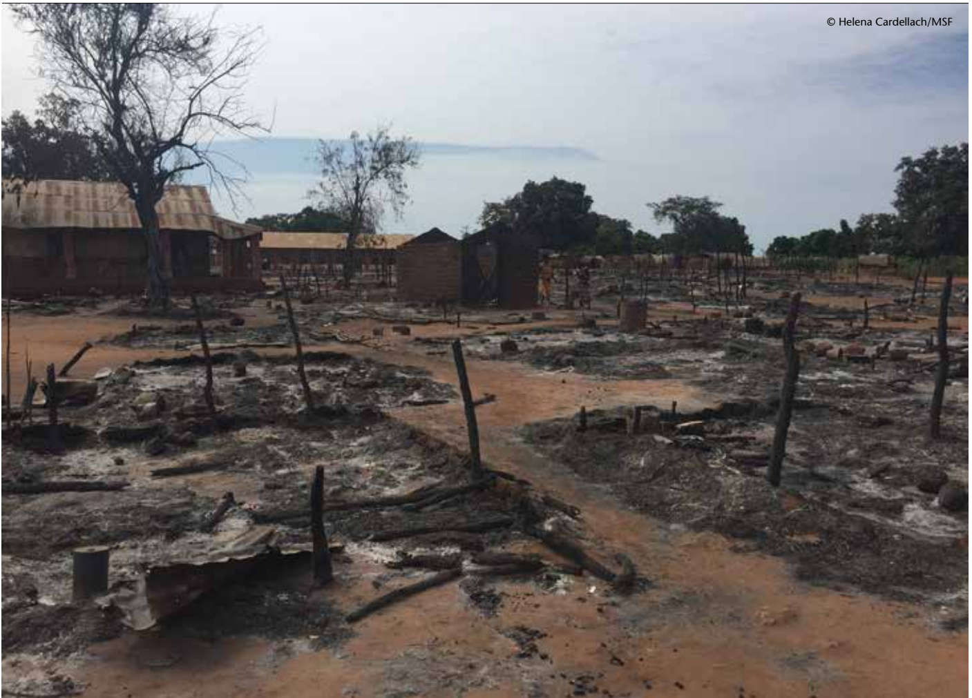
The remains of Batangafo village, Central African Republic, in November 2018, just over a week after violent clashes between armed groups.
