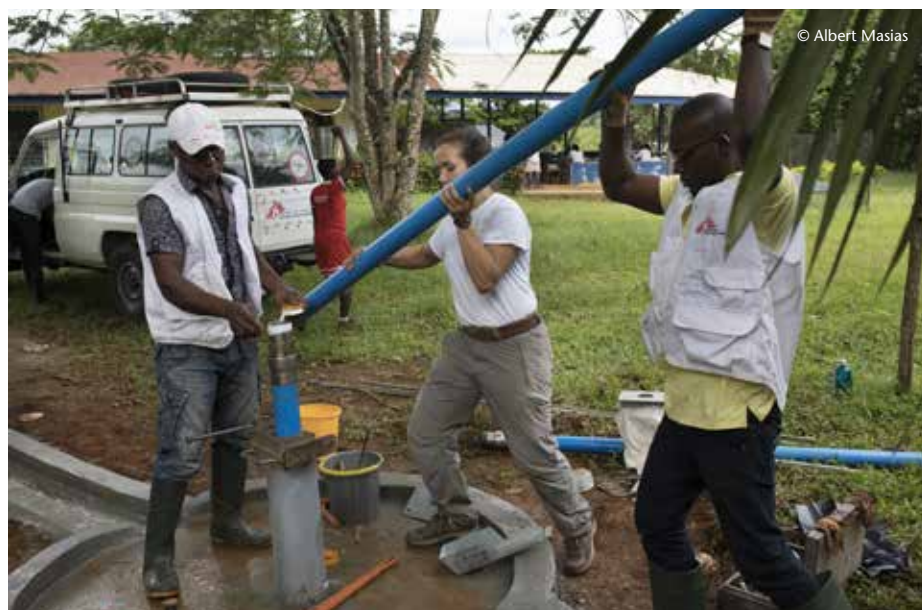
MSF water and sanitation experts install a hand-operated water pump at Abgokim clinic in Cross River state, Nigeria, November 2018.
