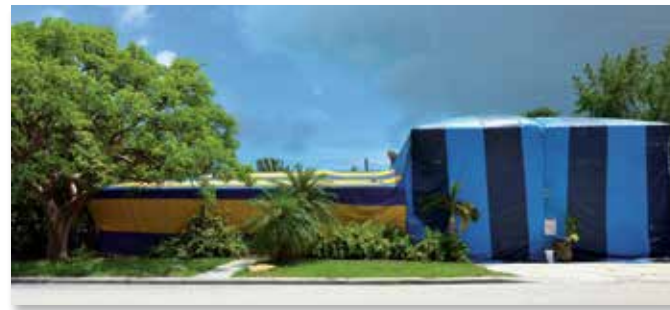
Structure being fumigated for pest treatment
