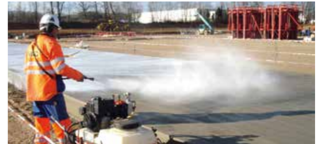
Immediate coverage or curing of concrete surfaces exposed to the elements is the most crucial step for protection of such surfaces.
