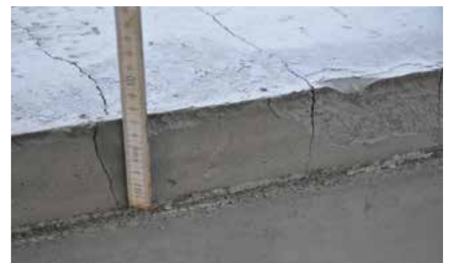
Cracks due to plastic shrinkage in a concrete pavement caused by insufficient surface protection prior to premature drying.
