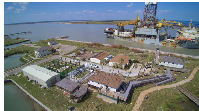
Damage to facilities at the Mission-Aransas National Estuarine Research Reserve following Hurricane Harvey.
