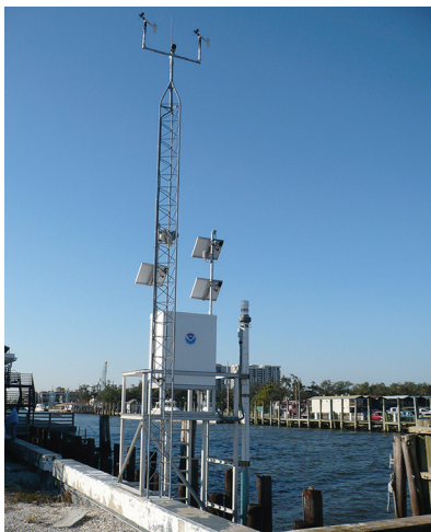
Elevated tide station with wind sensors. Credit: CO-OPS
