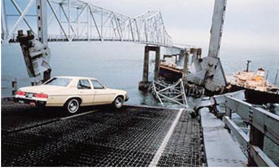
Scene from the Sunshine Skyway Bridge collapse in May, 1980. Credit: St. Petersburg Times
