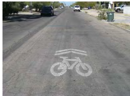
Bike Route with Shared Lane Marking
