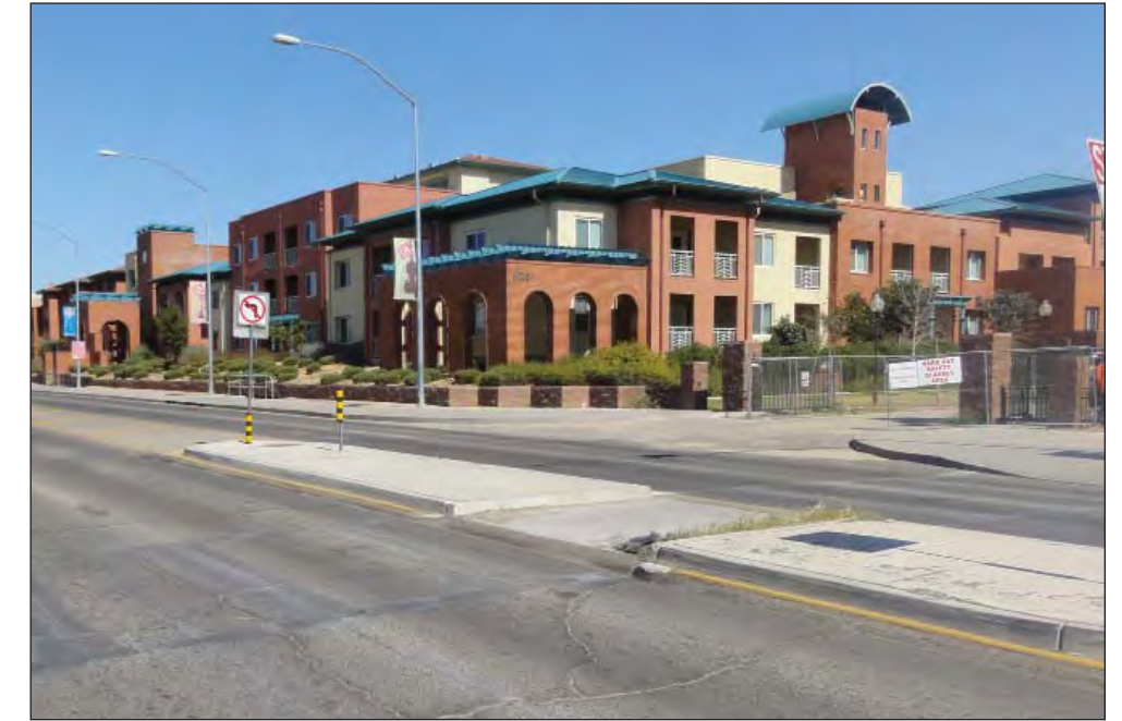
There is an existing pedestrian refuge island and traffic diverter on Euclid Avenue at 5th Street
