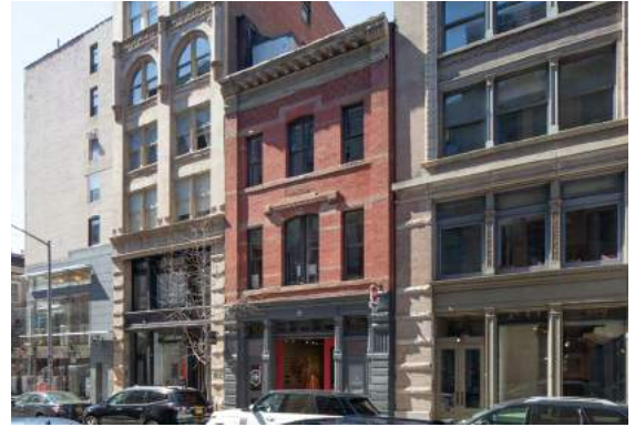
Figure 36. Gay Activists Alliance Firehouse, 99 Wooster Street, Manhattan. Photo by Christopher D. Brazee/ NYC LGBT Historic Sites Project, March 2016.
