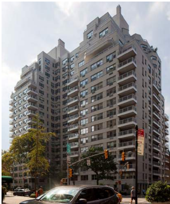
Figure 68. Larry Kramer Residence, 2 Fifth Avenue, Manhattan. Photo by Christopher D. Brazee/NYC LGBT Historic Sites Project, September 2016.
