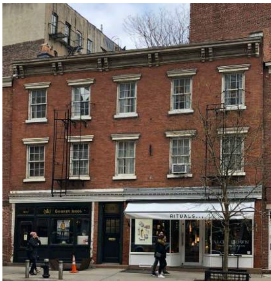
Figure 86. Lorraine Hansberry Residence, 337 Bleecker Street, Manhattan. Photo by Amanda Davis/NYC LGBT Historic Sites Project, March 2018.
