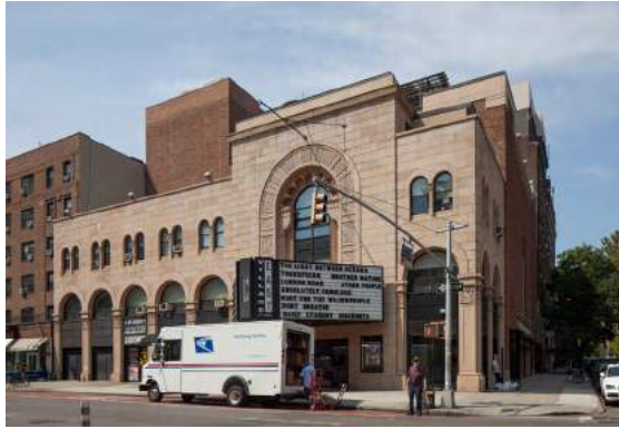
Figure 19. Louis N. Jaffe Art Theater / 181 Club / Phoenix Theater / Multiple Apartments, 181-189 Second Avenue, Manhattan. Photo by Christopher D. Brazee/NYC LGBT Historic Sites Project, September 2016.
