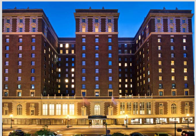
Top to bottom, left to right: A. Phillip Randolph Houses, Harlem; TWA Terminal, Queens; Richardson Olmsted Complex, Buffalo; Hotel Saranac, Saranac Lake; Hotel Syracuse, Syracuse
