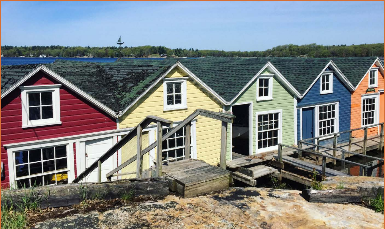
Five historic boathouses on Wellesley Island, Thousand Island Park, Jefferson County
