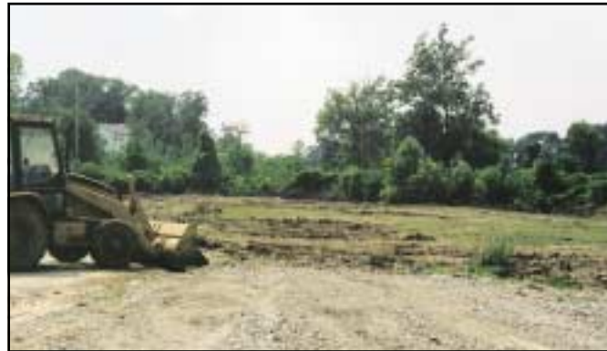
Ground preparation for a soccer field in Arnold.
