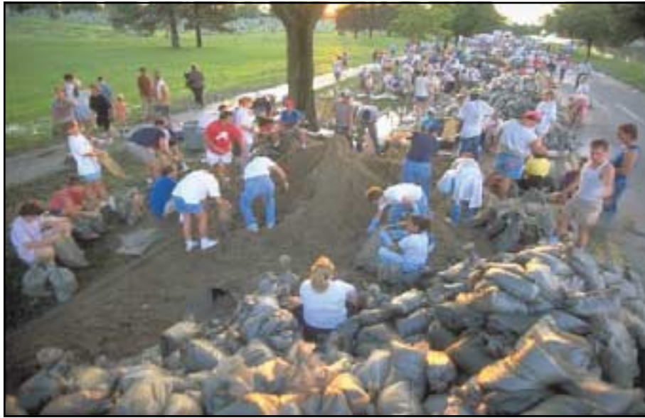
Volunteers performing sandbagging operations in St. Charles County.
