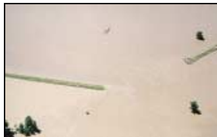
Broken flood control levee
