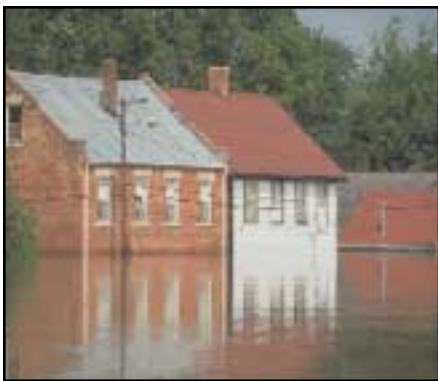
Extensive flooding in St. Genevieve.
