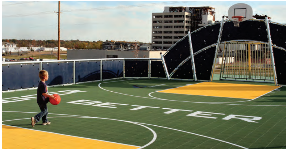
The new basketball court built in Cunningham Park, which was destroyed in the tornado. The destroyed St. John's Mercy Hospital is in the background.
