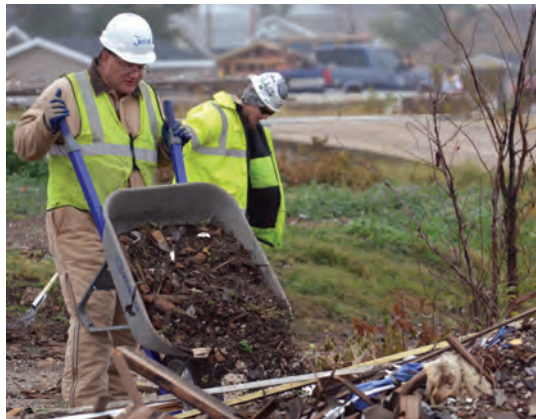
Disaster Recovery Jobs Program employees clear debris.
