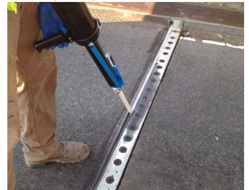
Sikasil®-728 RCS being applied to a horizontal joint
