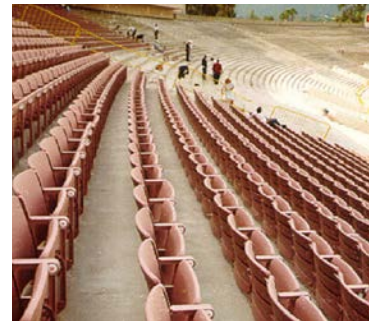
Sikadur® 55 SLV crack healer/sealer applied to seating area
