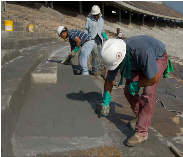
Spall repairs on a bleacher edge with SikaQuick® VOH
