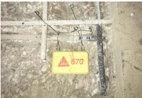
Sika® FerroGard® Anodes used to prevent corrosion of rebar in reinforced concrete
