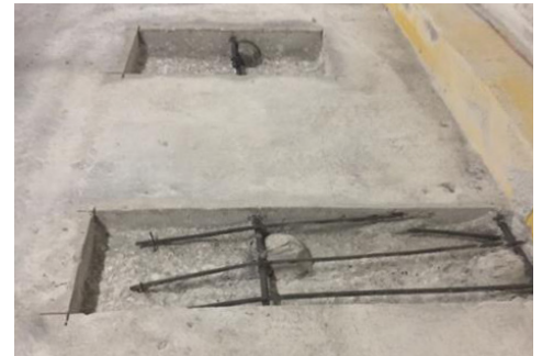
Sika® Repair mortar used to embed Sika® FerroGard® anodes
