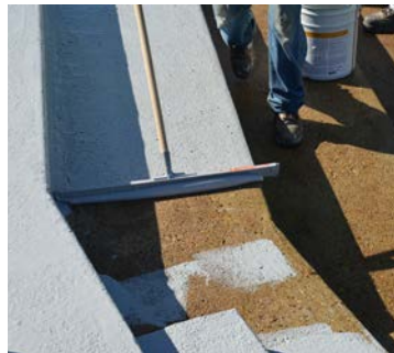
Sikalastic® 720 system application
