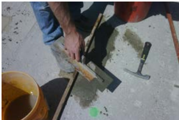
SEATING AREA REPAIR
