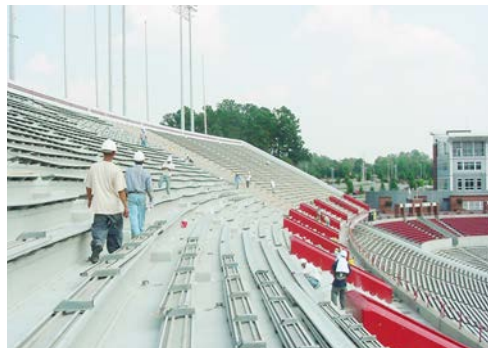
SikaTop® 144 applied onto the concrete structure underneath the bleacher seating
