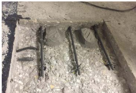
Sika® FerroGard® anodes installed onto an existing slab
