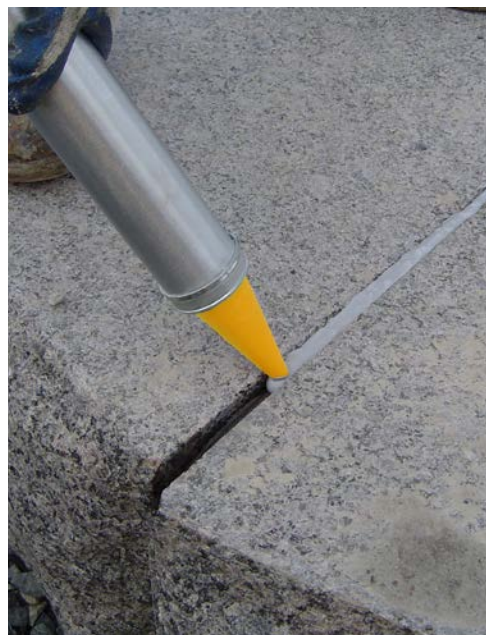
Sikaflex® 2c SL two component, self-leveling sealant applied to joints
