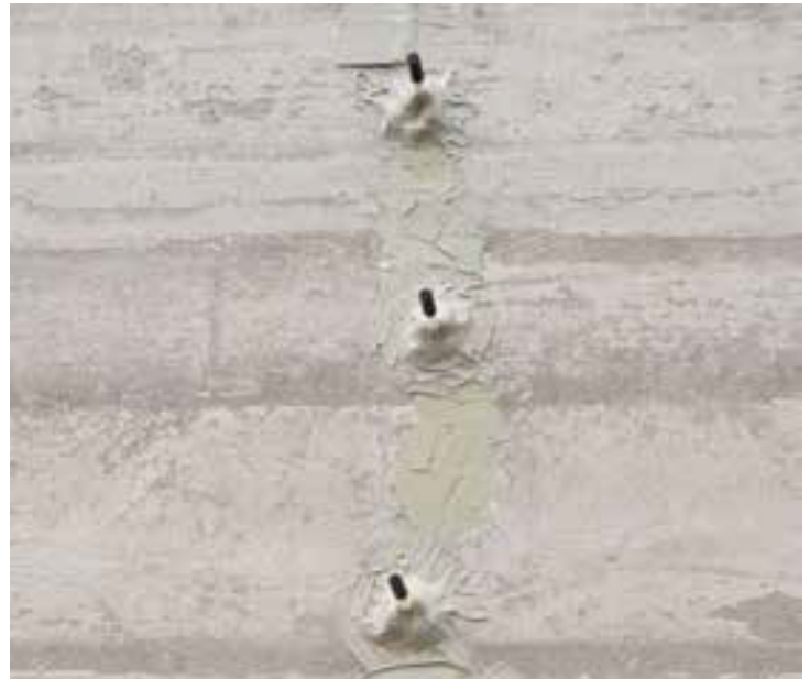
Cracks in concrete injected with ultra low-viscosity Sikadur® injection epoxy
