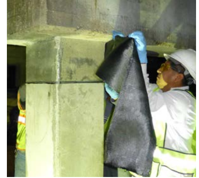
SikaWrap® PreSaturated 103C carbon fabric applied to column
