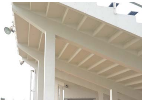
Sikagard® 670W coating applied onto an underside of a seating area
