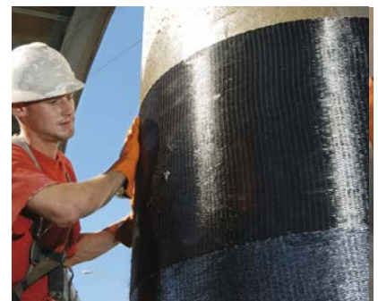
Strengthening concrete column with SikaWrap® fabric
