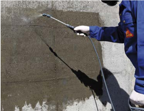
Application of Sika® FerroGard® 903
