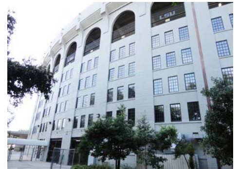
Sikagard® 670W acrylic protective coating spray applied over SikaTop® 144 on the north side of LSU Tiger Stadium
