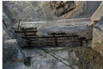
UNDERSIDE SPALLING
