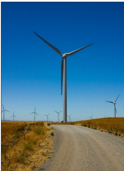
Figure 9. Wind turbine access roads can account for 38%–41% of nonusable land within a wind energy project's footprint (Diffendorfer and Compton 2014). Photo by Dale Carlson
