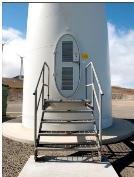
Figure 19. Locking door and warning signs on a wind turbine entrance. Photo by Travis
