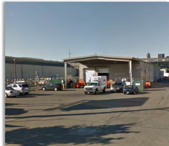
Amtrak's Food and Beverage Commissary at 222 South Holgate Street - Seattle
