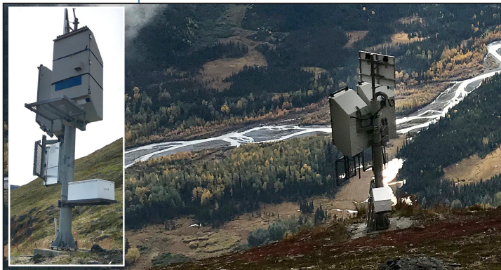
A type of RACS, the Blaster Box above 43 Mile path allows for remote avalanche mitigation at any time. Over the next several years, RACS will replace howitzers at avalanche control sites.
