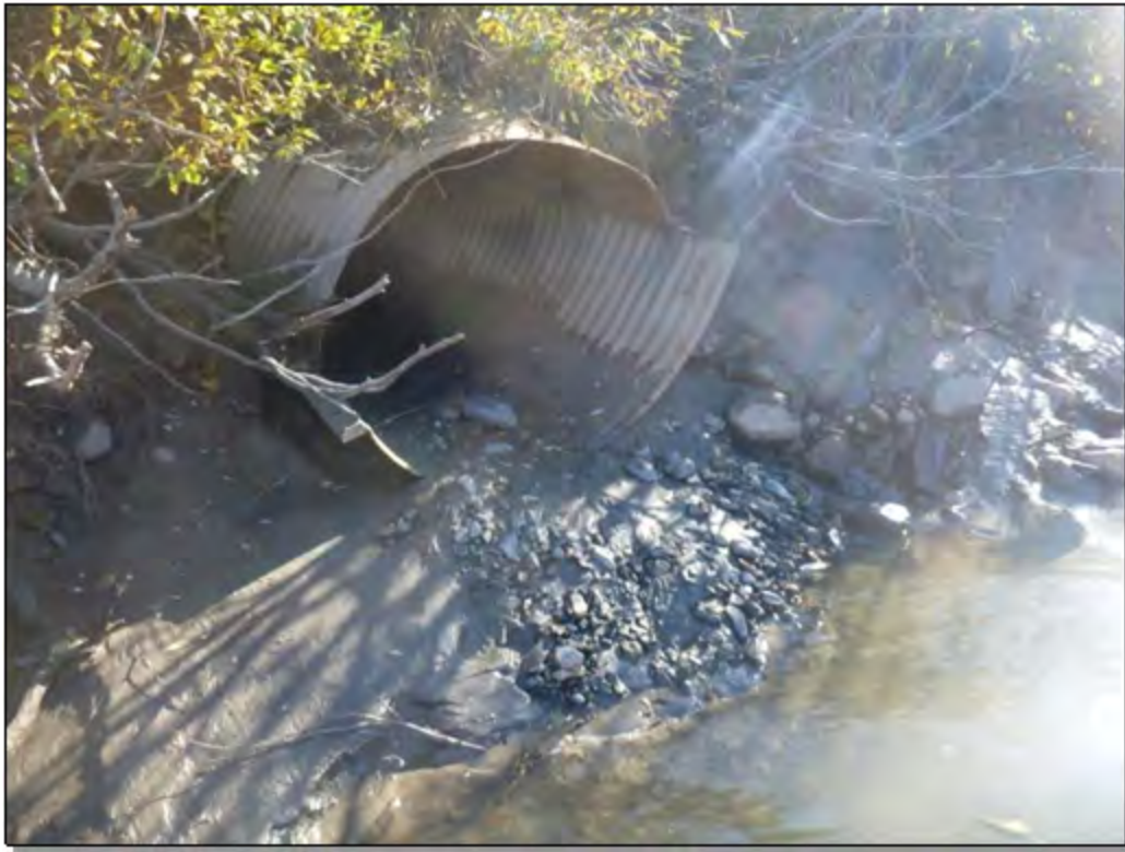
Site 15: South culvert. Photo taken September 29, 2016
