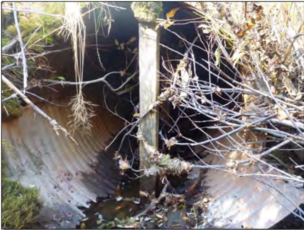
Site 9: Culvert. Photo taken September 29, 2016
