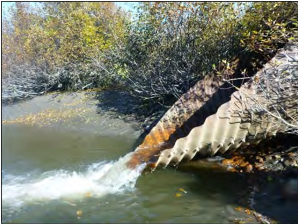
Site 15: North culvert. Photo taken September 29, 2016
