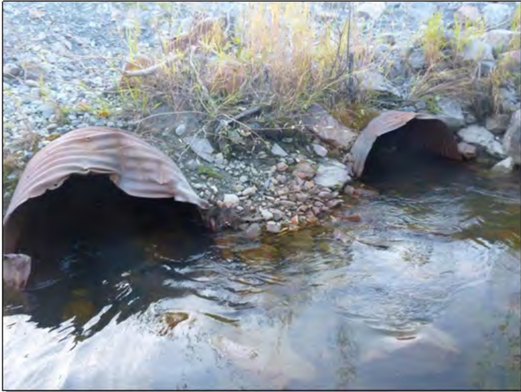
Site 43: Culvert. Photo taken September 29, 2016
