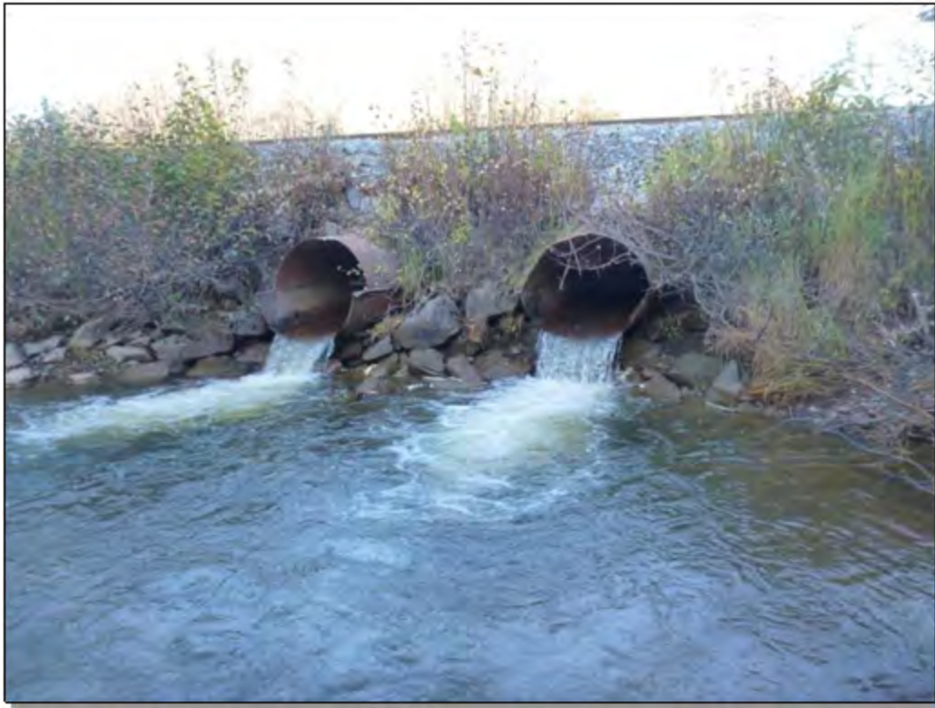
Site 41: Culvert. Photo taken September 29, 2016
