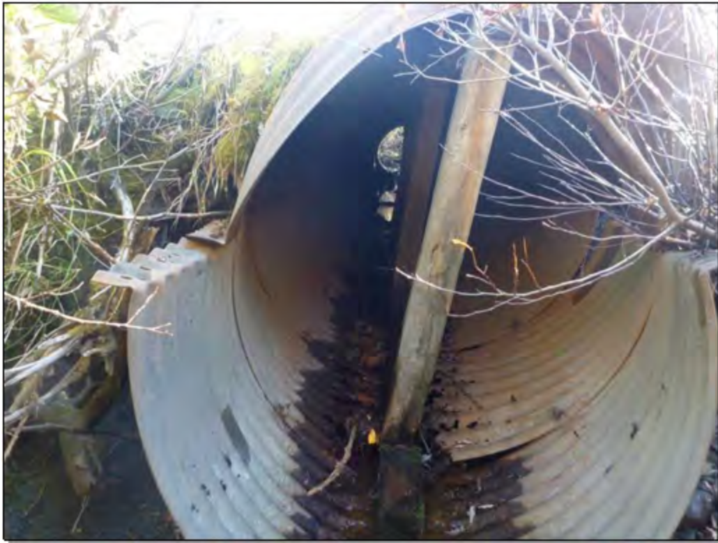
Site 10: Culvert. Photo taken September 29, 2016
