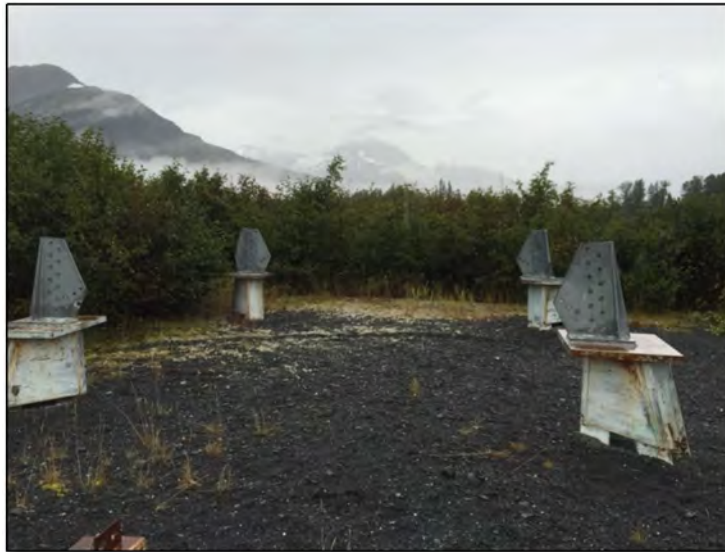
Inset 1. Abandoned microwave tower pad. September 6, 2016.
