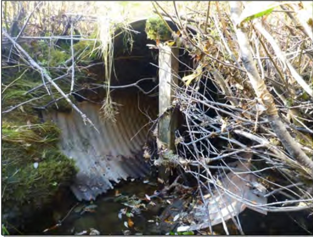
Site 9: Culvert. Photo taken September 29, 2016
