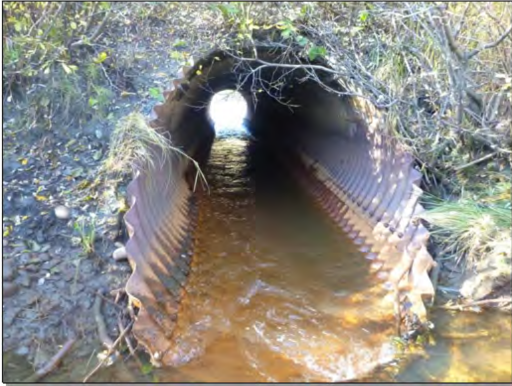
Site 16: Culvert. Photo taken September 29, 2016
