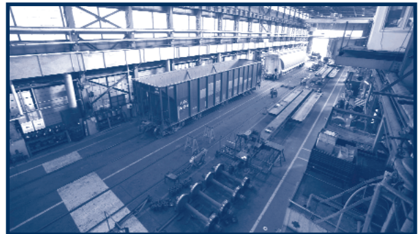
Anchorage Rail Yard Car Shop.
