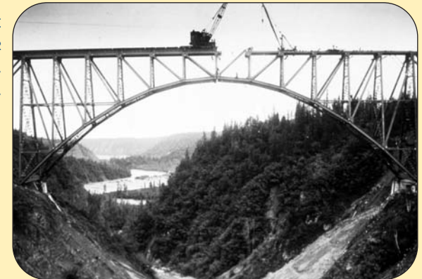
HURRICANE BRIDGE UNDER CONSTRUCTION. CIRCA 1921.
