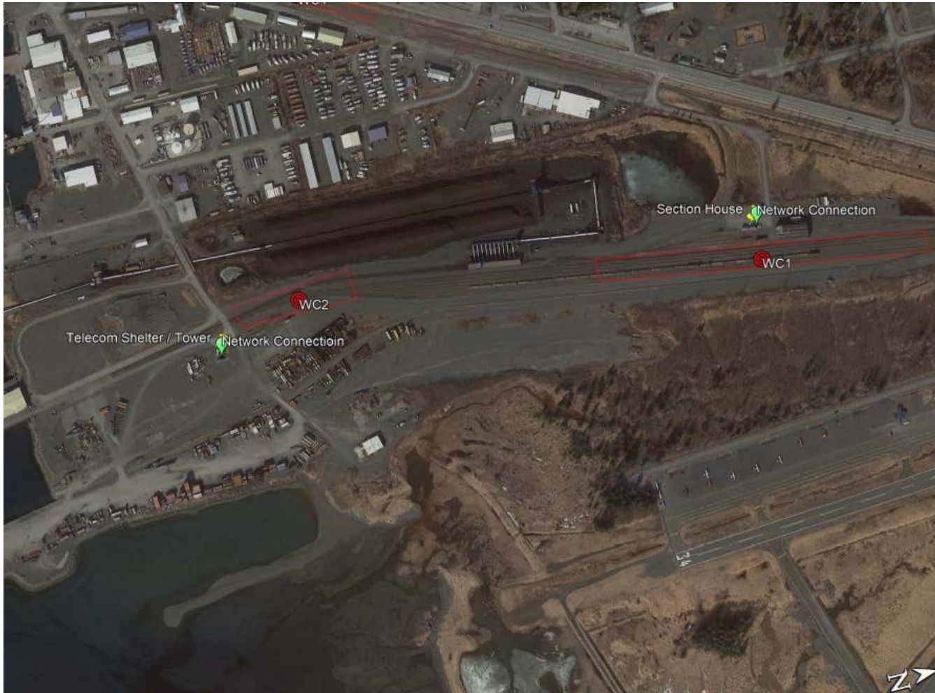
Telecom Shelter/Tower and Section House
