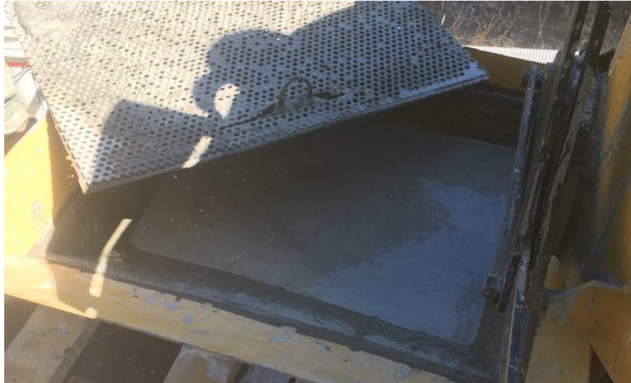
Figure 2.2: Grout consistency prior to installation
