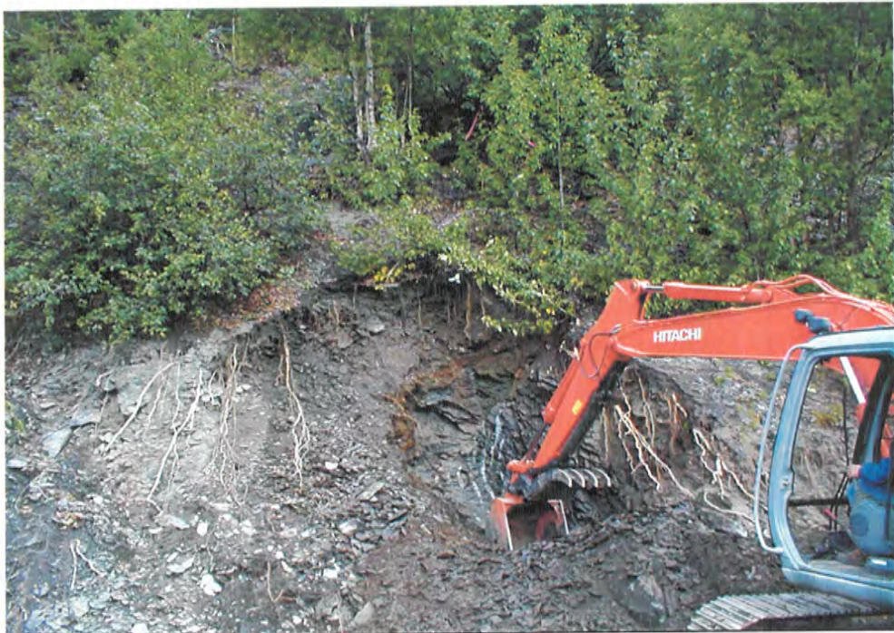
Excavator at Test Pit 13 near Abutment No. 5.
