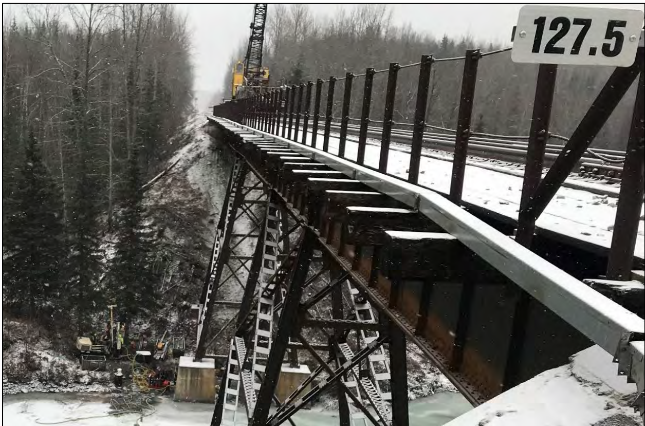
PHOTO: Drilling of Exploration B3 at north pier site of Bridge 127.5
