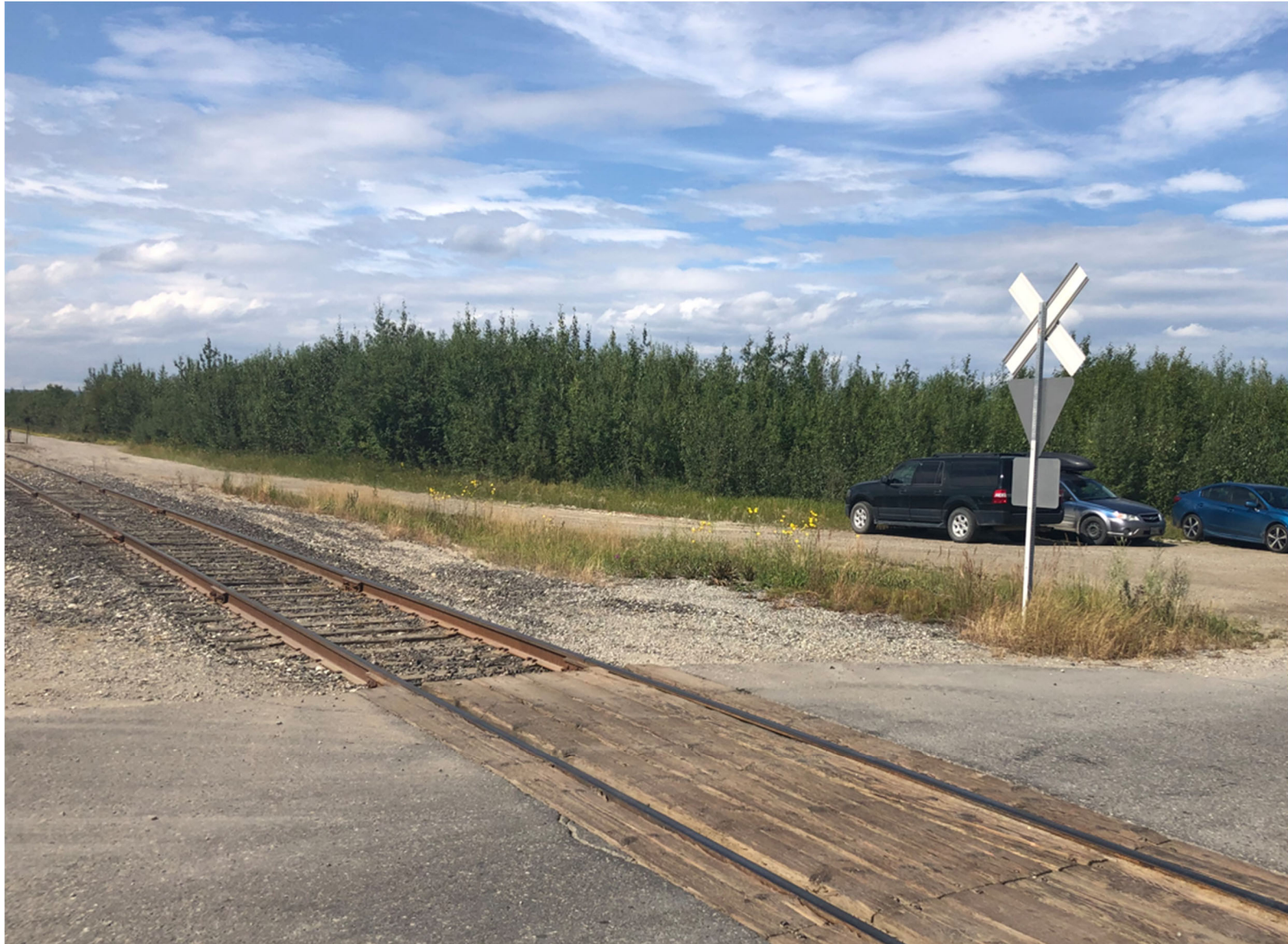
Figure 4 - Joints on West Side (July 2021)
