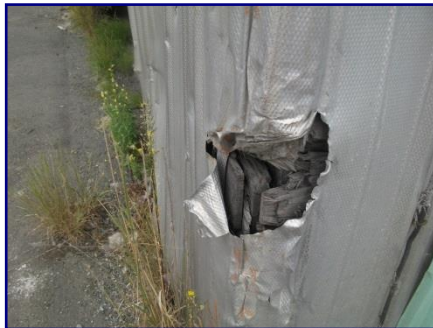
Exterior Felt under Siding
