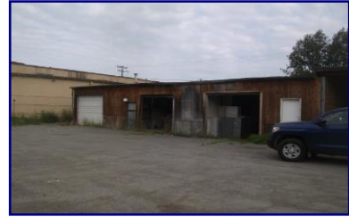
Back of Building
