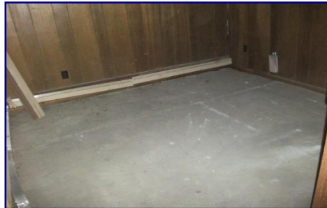
Unit 7 Office Area Tile
