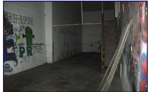
Unit A Last Bay
