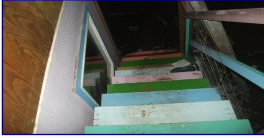
Unit C Stair case
